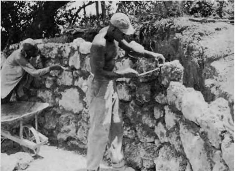
One of the retaining walls that was built in Officers' Country. ▶
