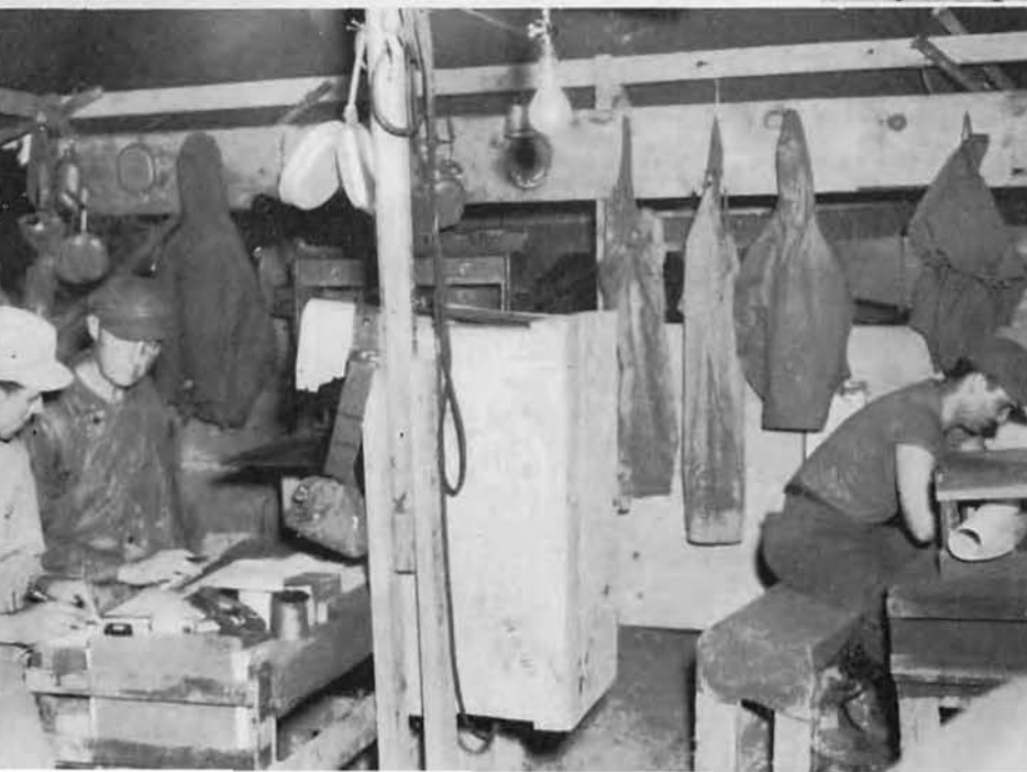
◀ The temporary Building Division Office. The planning and erection of all structures was controlled by this office. Shown in this picture from left to right are: A. DONATTO, SF3c, D. WILKINSON, CCM, and Julian A. OTT, Ensign, (CEC) USNR.
