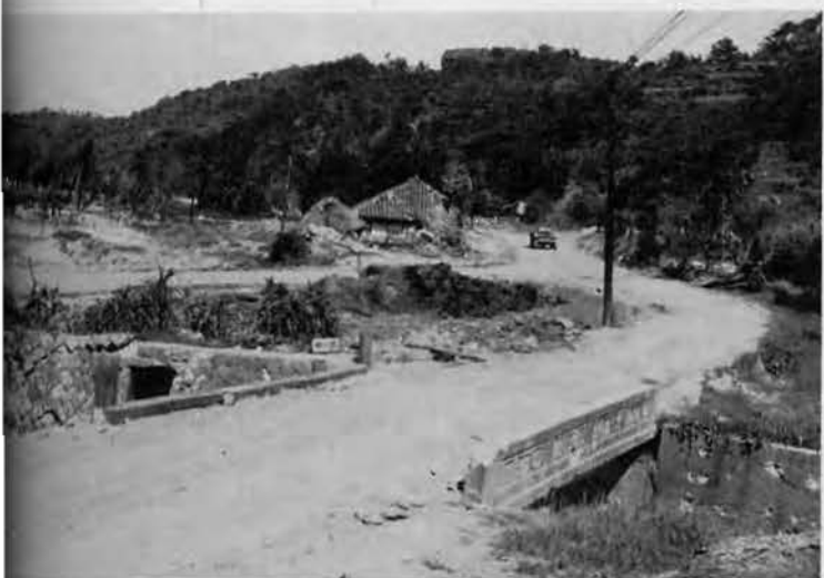
Yes, it is the same bridge or location rather, but a few hours of Seabee labor and ingenuity produced a bridge capable of supporting our heaviest vehicles. Note the hand work in the rock retaining wall to the left, which was built by Okinawans.
