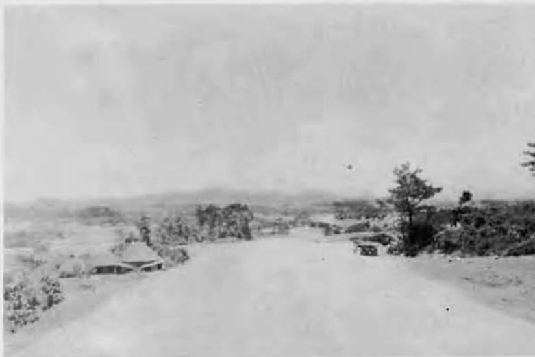
A finished product. A few days before, this would have been a wagon trail, but now a four lane, coral surfaced super-highway.
