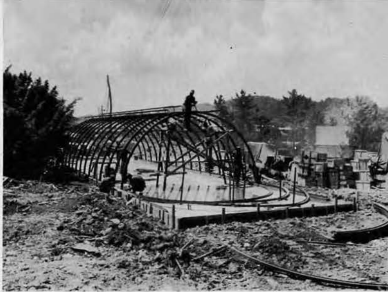
Erection of ribs on Chiefs' Mess. For some reason, which has never yet been brought to life, this building was constructed in record time. In fact it was going up so fast, work had to be suspended from time to time.
