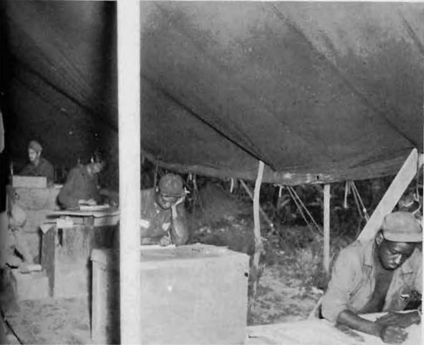
◀ The temporary Engineering Office. This hurriedly erected structure served to house the draftsmen while designing and drawing plans for future jobs. Shown in the picture from left to right are: R. G. RAMSEY, CM1c, F. L. SNYDER, CCM, (kneeling), W. TAYLOR, CM2c, S. HOWARD, CM2c, and T. McCULLOUGH, SF2c.
