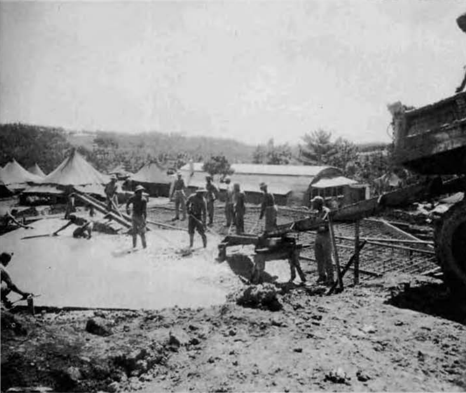
◀ Pouring concrete foundation for 126,000 gallon Raw Water Storage Tank.
