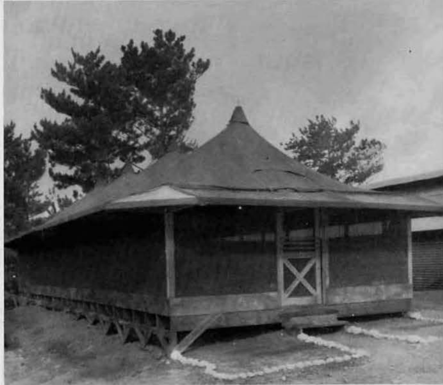
Close-up view of Sick Bay Ward. Frame 16'x50' covered with tent. We were very fortunate in having a minimum number of patients to patronize this room. ▶
