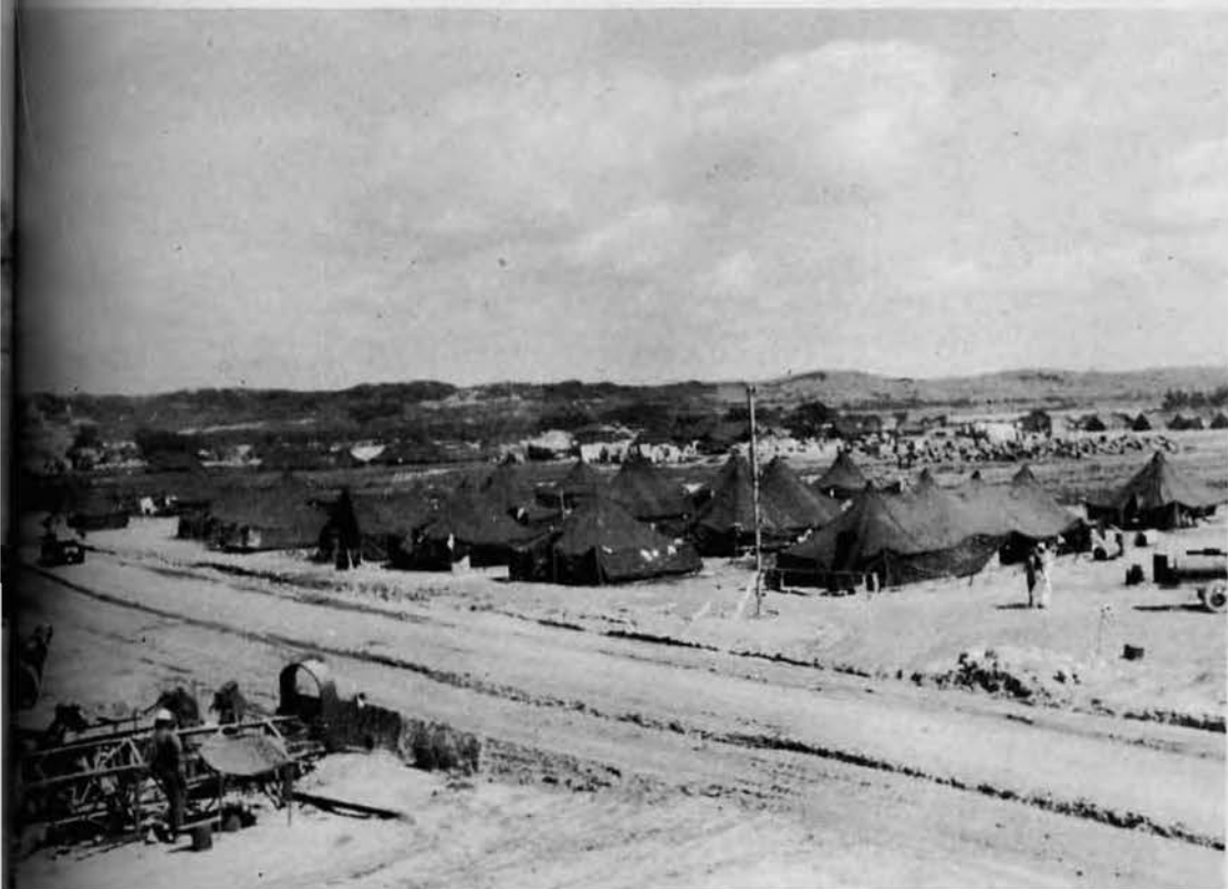
A small detached unit remained on the beach to handle and guard supplies and equipment as it came ashore. Their camp can be seen in the center foreground.
